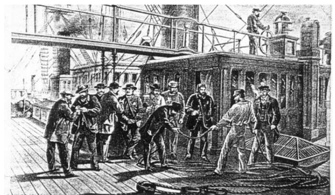
**Fig. 2 Searching for a Fault in a Recovered Length of the First Operational Transatlantic Cable in 1868**
