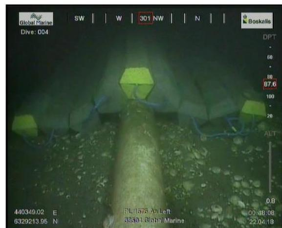
**Figure 1.5: 300m Mattress (exposed pipeline)**
