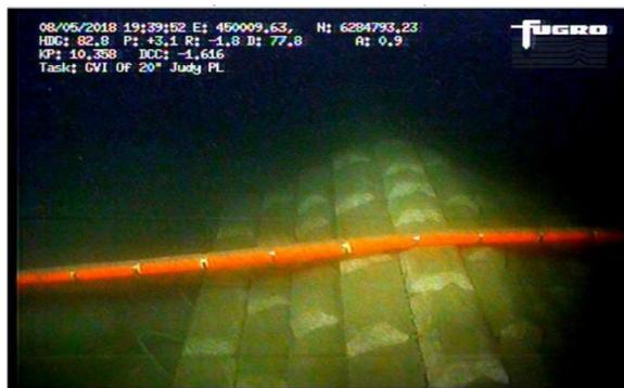
Figure 1.1: Cable Suspension
