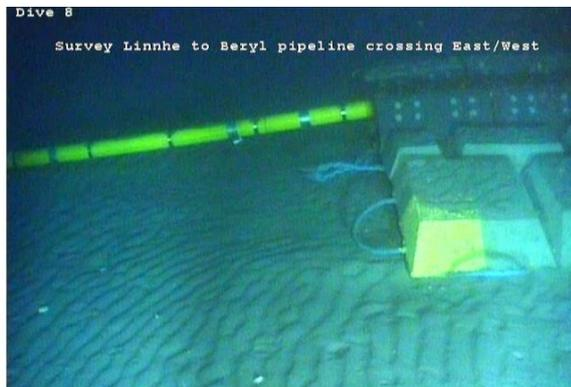
**Figure 1.3: 300m Mattress (buried pipeline)**
